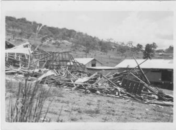
Hospital Wards – Murray Barracks.
