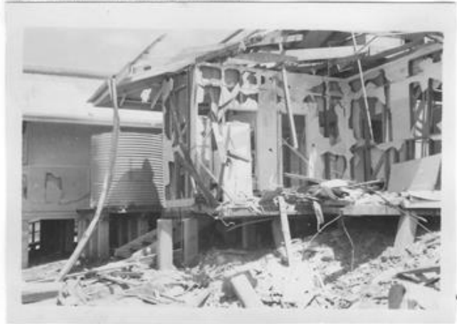
Hospital Theatre – Murray Barracks.
